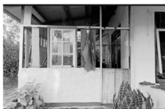
Figure 4. The TBM Keik Tsinagi occupies an ancillary room constructed adjacent to the main residence.
